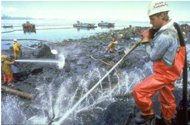
Figure 8.4 Cleanup workers spray oil-covered rocks on Prince William Sound with high-pressure hoses. (Photo Courtesy of Exxon Valdez Spill Trustee Council)
