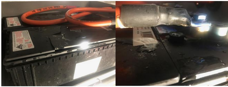
Figure 13. Batteries in this installation are separate from the switchgear. Wiring is routed through the panel via watertight/gastight glands. The door has ventilation. All components are labelled.
