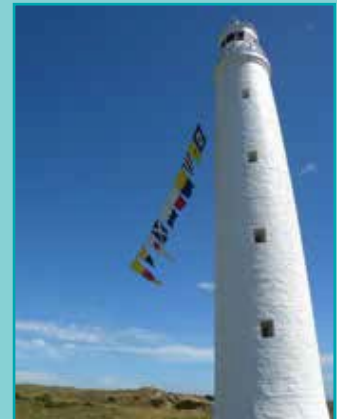
Figure 61. Cape Wickham Lighthouse. Photo source: AMSA, 2011
