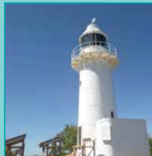
Figure 6. Cape Leveque Lighthouse Photo source: AMSA 2020
