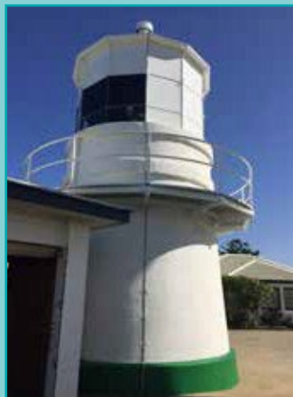
Figure 20. Nobby's Head Lighthouse Photo source: AMSA, 2019
