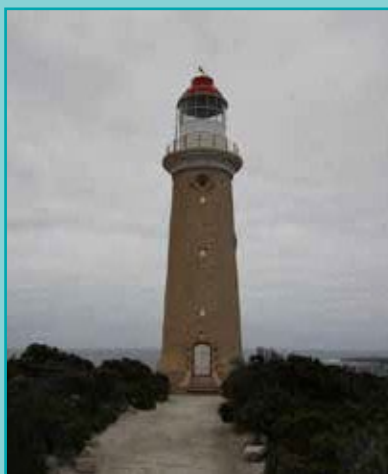
Figure 92. Cape du Couedic Lighthouse. Photo source: AMSA, 2015
