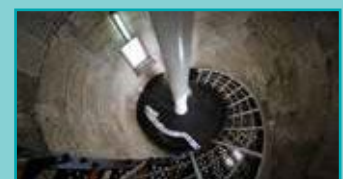
Figure 5. Cape Leeuwin Lighthouse Photo source: AMSA, 2015
