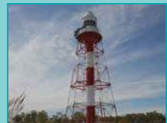
Figure 52. Charles Point Lighthouse. Photo source: AMSA, 2015
