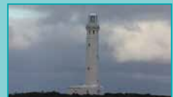
Figure 3. Cape Leeuwin Lighthouse Photo source: AMSA 2019
