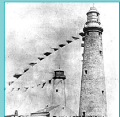
Figure 18. Rottnest Island Lighthouse. Image courtesy of the National Archives of Australia. NAA: A6247, A22/2 (© Commonwealth of Australia (National Archives of Australia))
