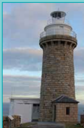
Figure 48. Wilsons Promontory lighthouse. Image courtesy of the National Archives of Australia. NAA: A9568, 6/9/1 (© Commonwealth of Australia (National Archives of Australia))
