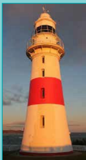
Figure 77. Low Head Lighthouse. Photo source: AMSA, 2016
