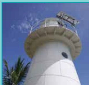
Figure 79. Dent Island Lighthouse. Photo source: AMSA, 2018
