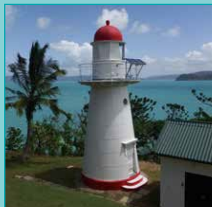
Figure 80. Dent Island Lighthouse. Photo source: AMSA, 2018
